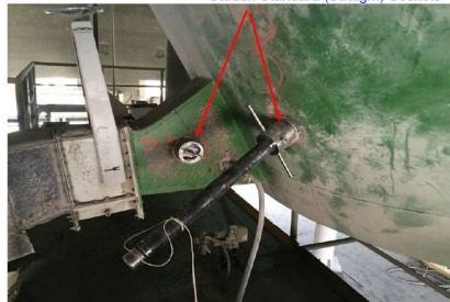
CARDOX TUBES Applied around discharge area of silo
